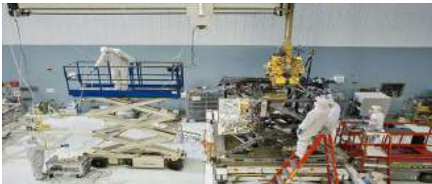
Fig 2.6:- NIRCAM being installed into the instrument module
